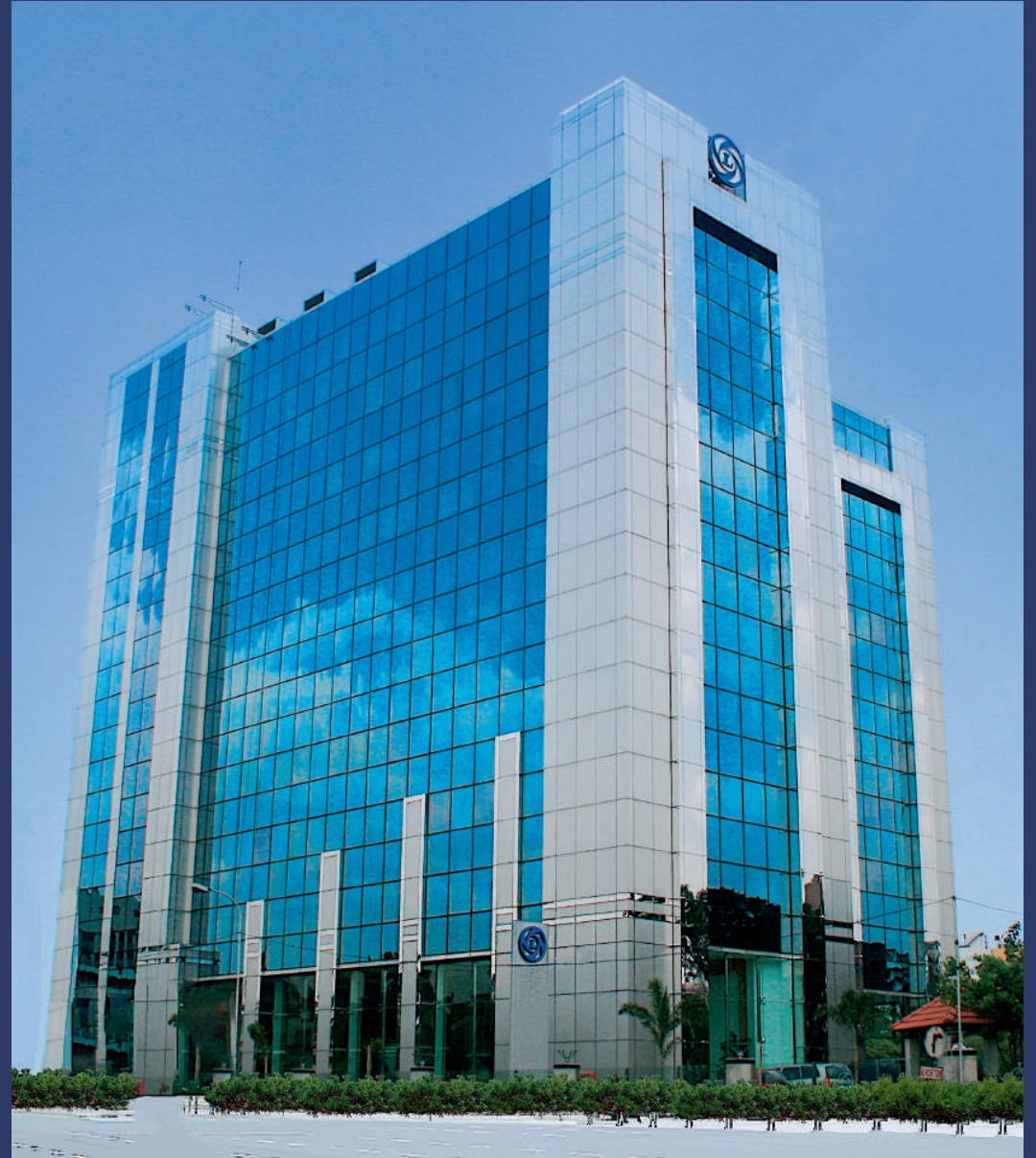
Ashok Leyland HQ, the first project outfitted with HYGREE Modular Toilet Solutions
